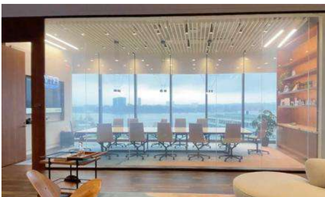
Light at an angle towards the smart glass or excessive light from the outdoors
